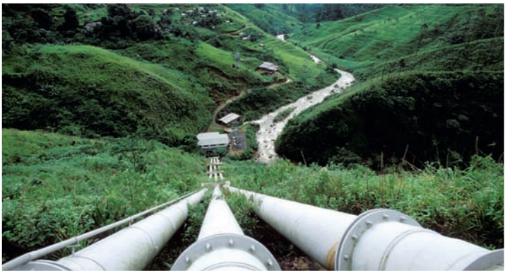
Water pipes at mini hydroelectric plant
