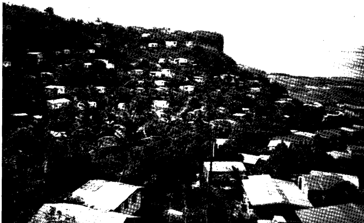
Fig. 39. Project No. 11: a view of the squatted area of Muller Village.
