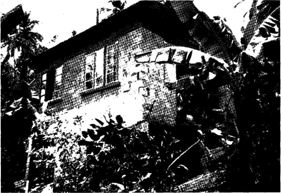
Fig. 15. Building materials typically used in Dominica today: cement, blocks, galvanized roofing, glass windows.
