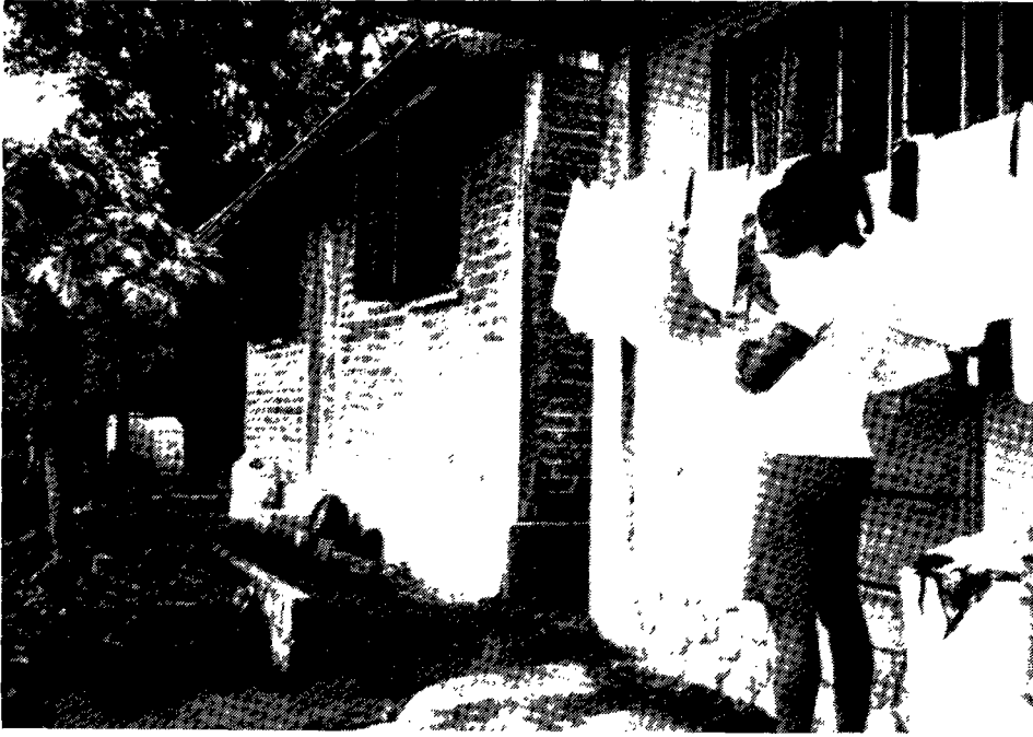
Fig. 19. Bricks used exceptionally for this house: the corners are cement pillars.
