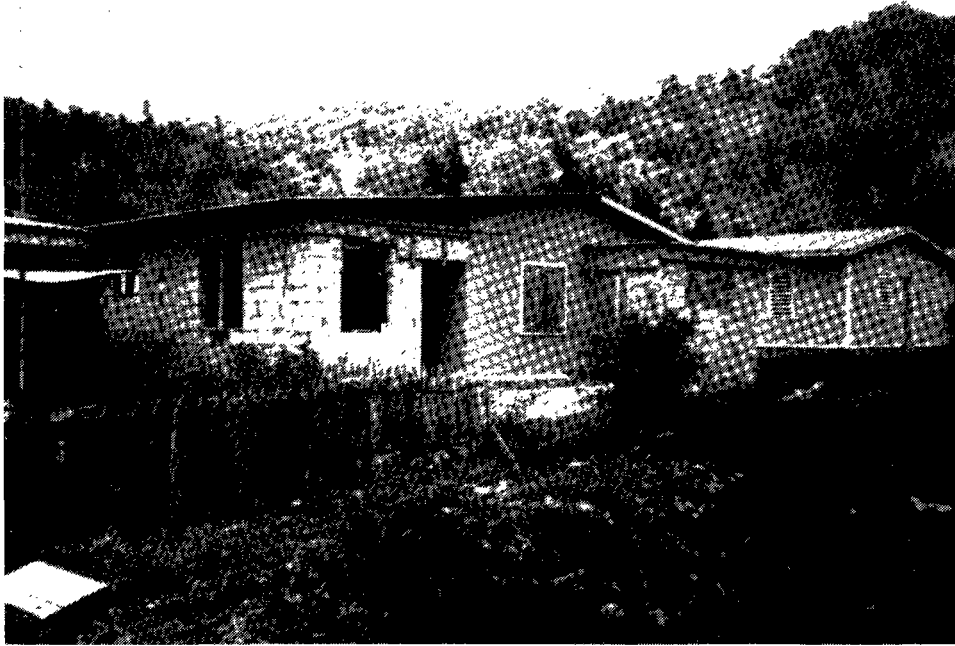
Fig. 21. Project No. 1. Bath Estate houses.
