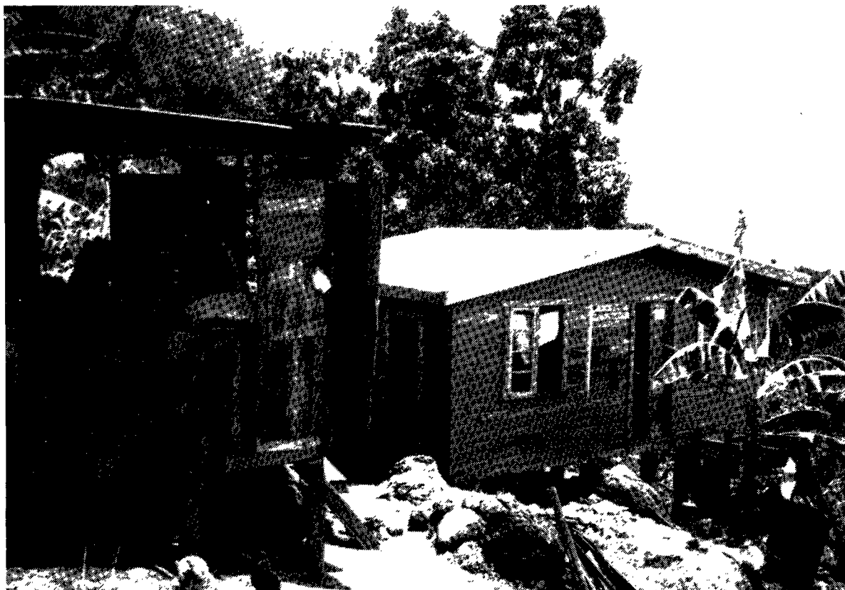
Fig. 42. Project No. 15: Rebuilding by self-help.
