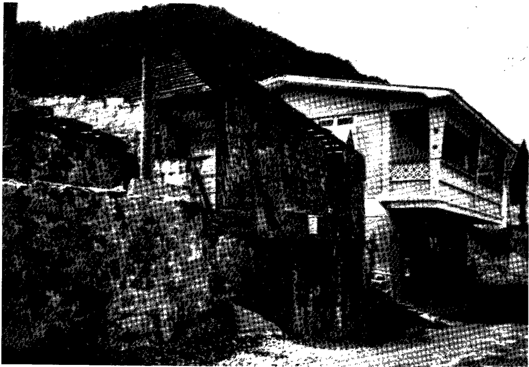
Fig. 3. House destroyed by hurricane David.
