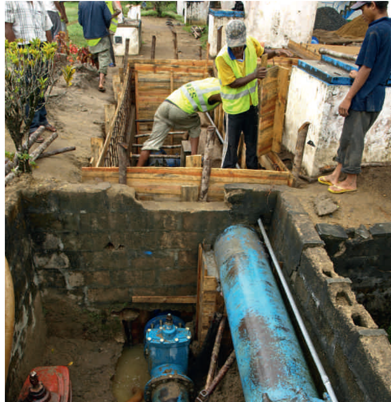
Fitting pipes for a water distribution system in Madagascar.
