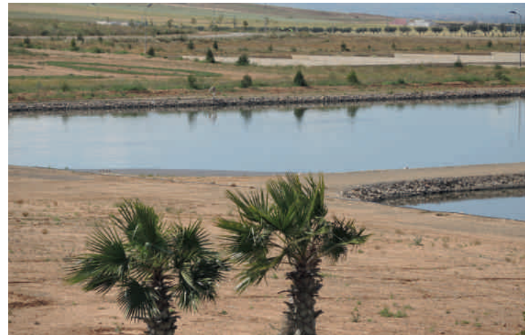
Water Purification Plant in Oujda, Kingdom of Morocco.
