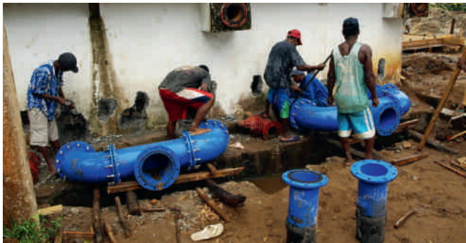
Works on a double layer filter in Madagascar.
