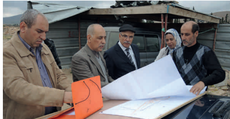
Technicians and local authorities overseeing the building site for a new purification plant in the region of Oriental, Kingdom of Morocco (2013).
