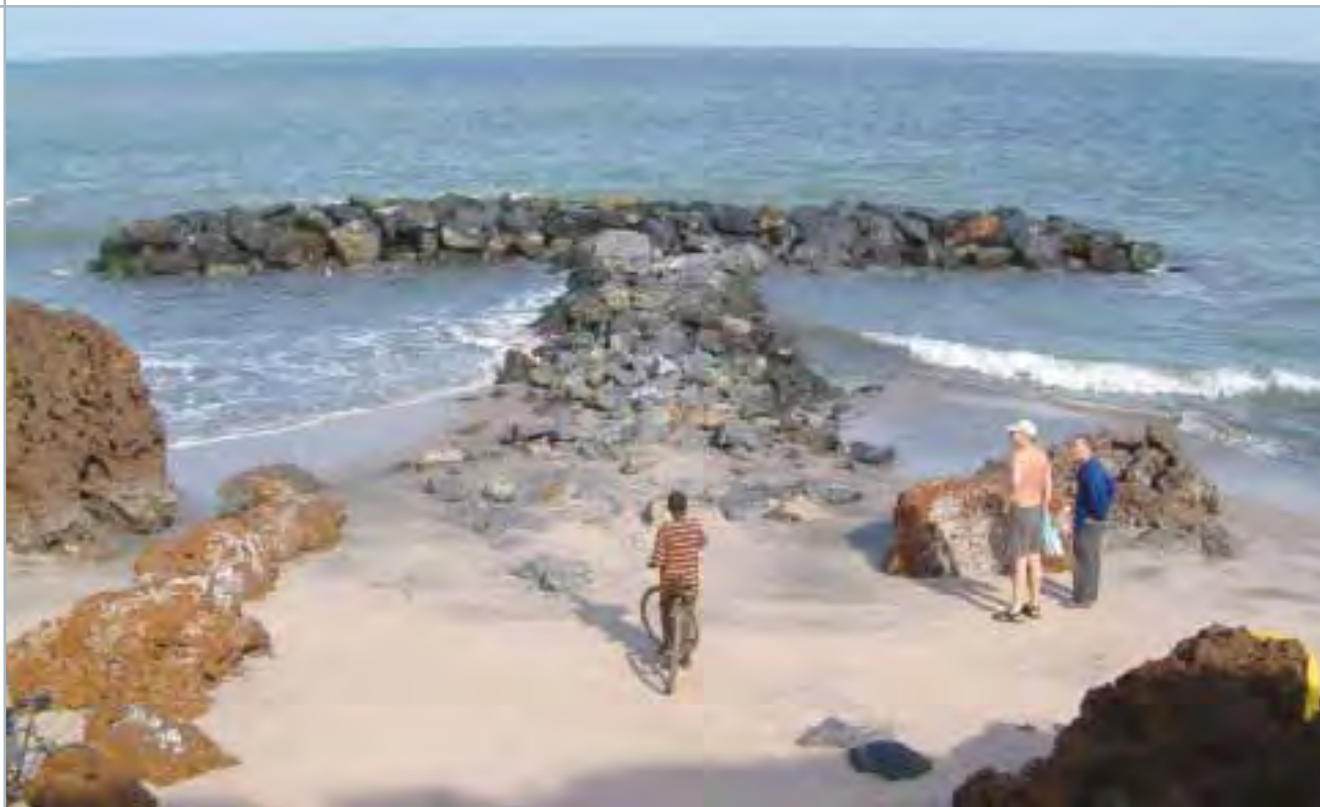
▲ A T-shaped groyne made of sea rock, backed by a newly restored sand beach, will protect this part of the coast for a long time.
